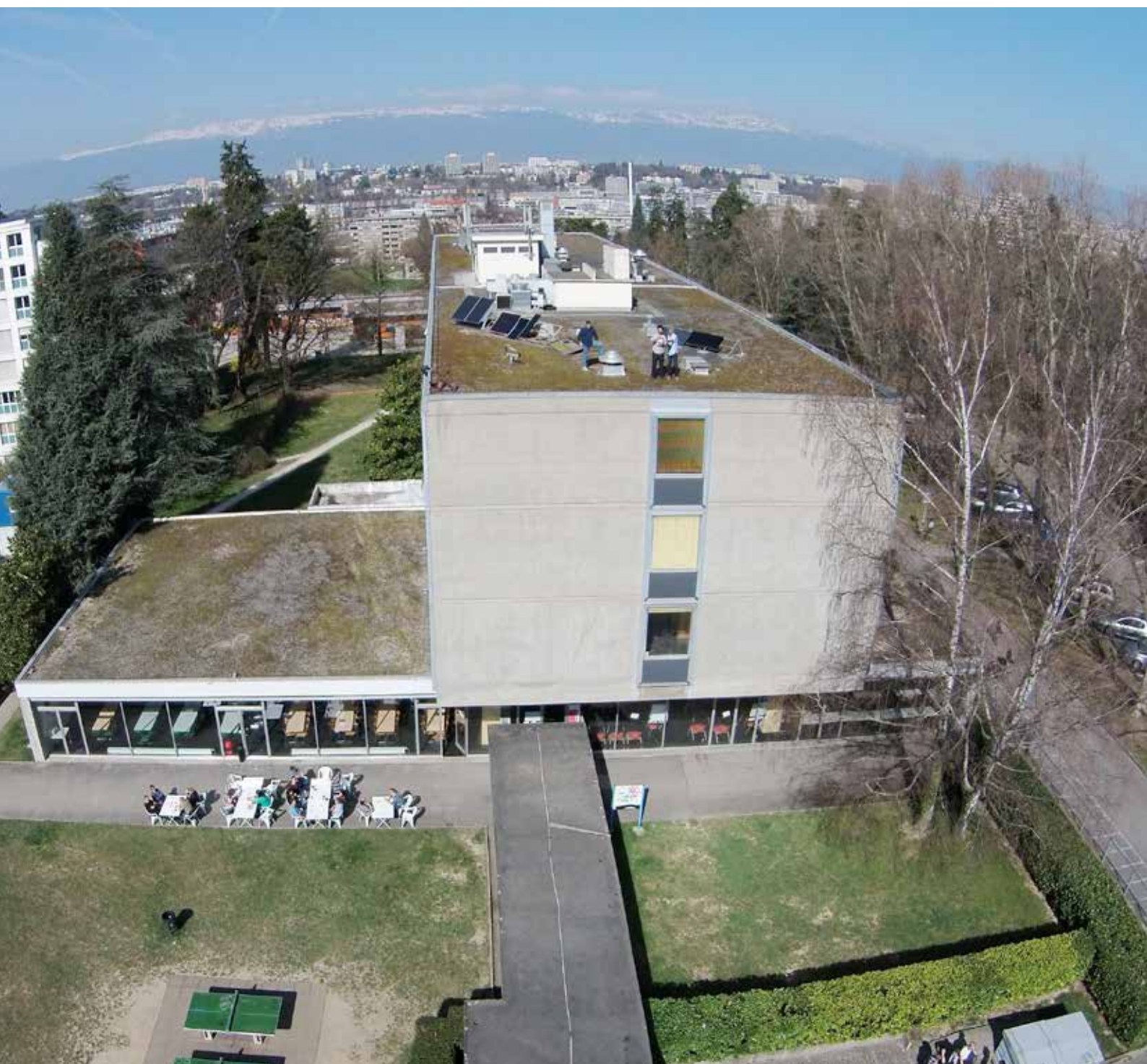
Battelle building A drone view, March 19 th 2014.
